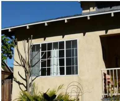
**Not this: mullions were removed and flush window was installed instead of recessed**
