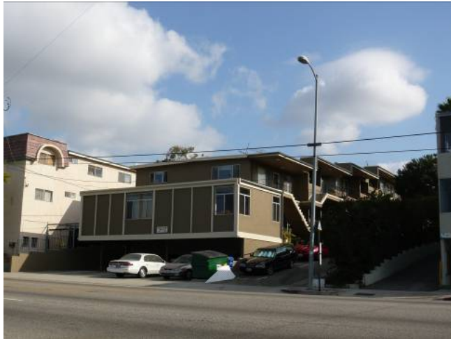
Building steps up as the site slopes up
