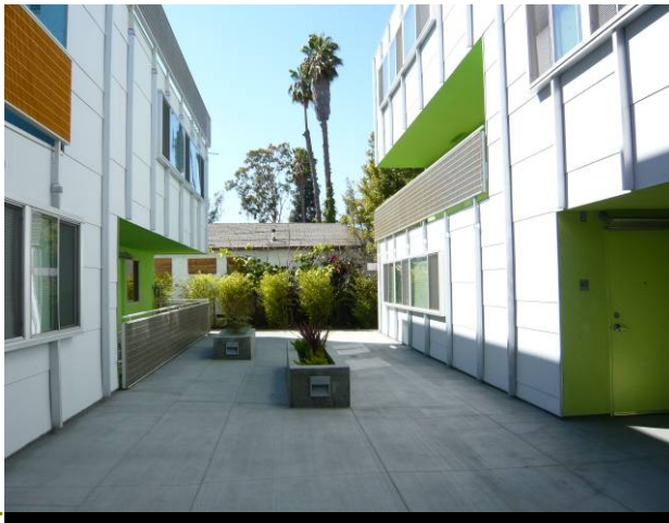
Building design is reinforced with color, material and detail
