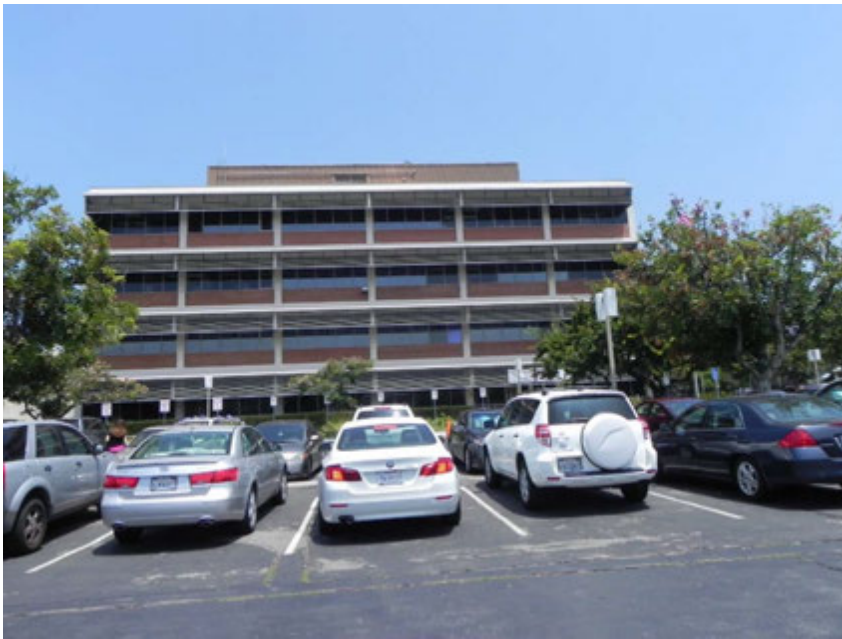
South (primary) façade of the 1971 administration building looking north from the parking lot.
