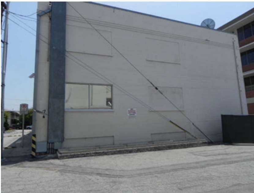
West façade of the 1938 warehouse building looking east from alley.
