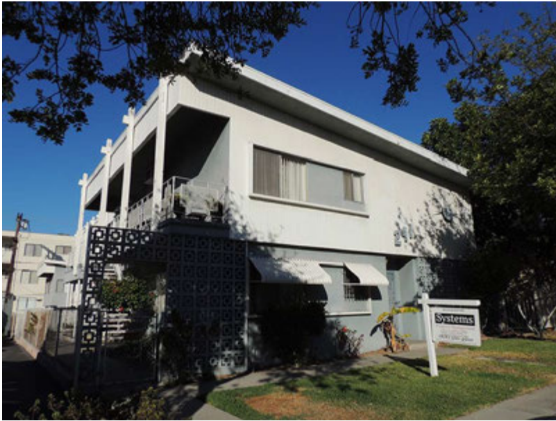
East façade of the apartment building looking northwest from N. Jackson Street.
