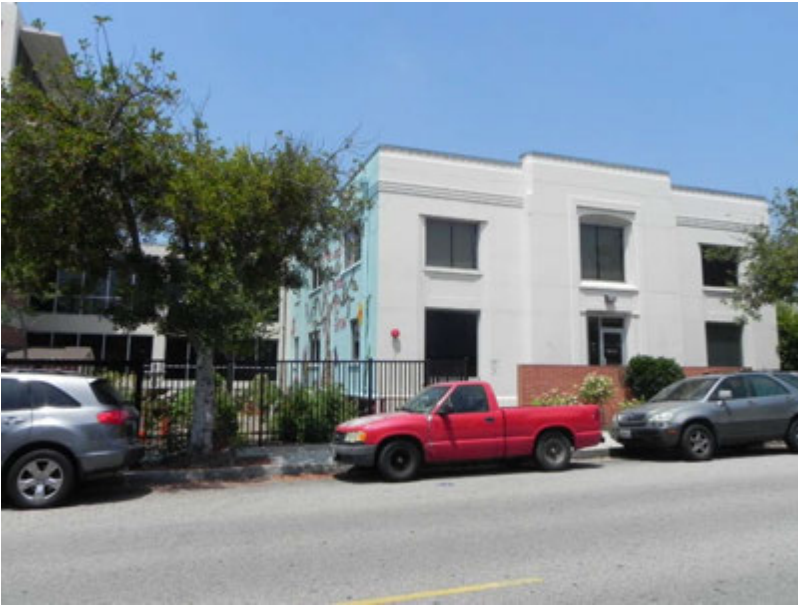
East (primary) façade of the 1938 warehouse building looking west from N. Jackson Street.
