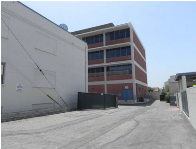
Looking south from alley to north façade of the 1971 administration building.
