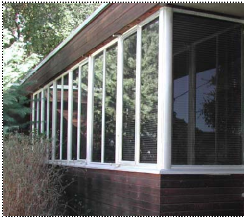
Above: Both the metal casements and the horizontal banding of these windows are characteristic of Modernism.
