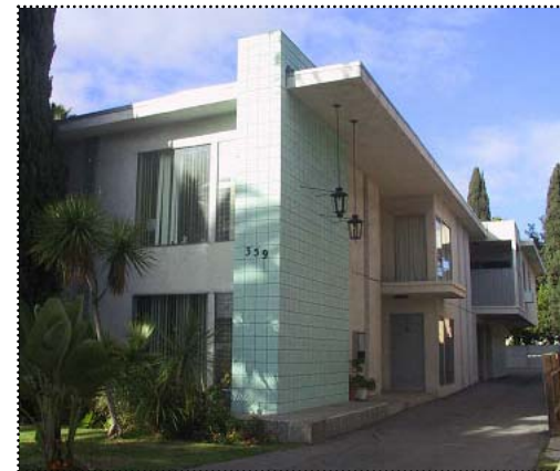
Below: The intersecting roof and wall planes of this apartment building are character-defining features. Polished stone mosaic creates the blue finish.
