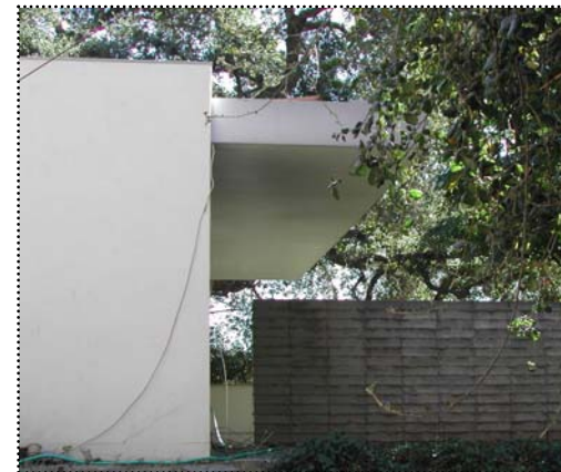
Above: This porch is recessed behind a row of simple posts and beneath the flat roof. Below: A simple cantilevered canopy can substitute for a traditional porch.
