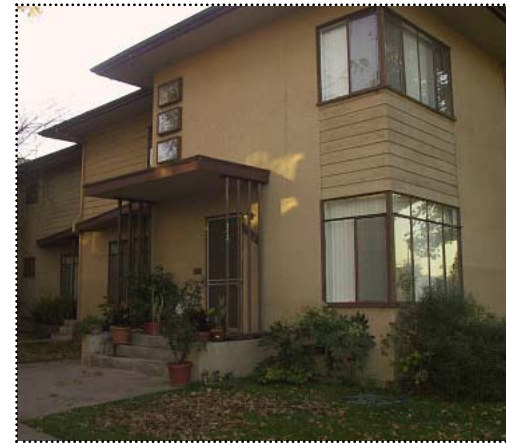
Above: This apartment building, while traditional in form, exhibits the influence of Modernism in its steel casement windows and its clean lines.
