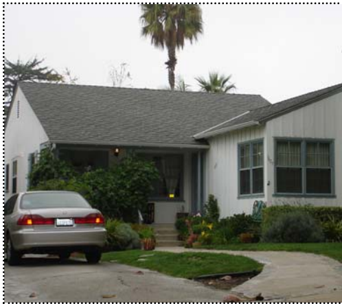
Above: This roof has a primary side gable with a prominent front-facing cross gable.
