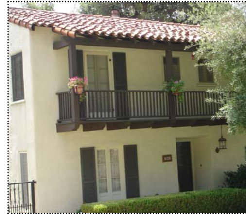
Above: Smooth stucco cladding is a common attribute of the Monterey style.
