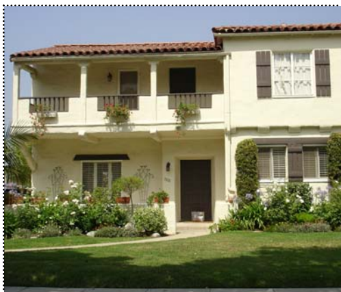
Below: This house is characteristic of the style in plan and height. As part of its L-shaped plan, the balcony is incorporated beneath the main roof, and the first floor is slightly recessed below it.
