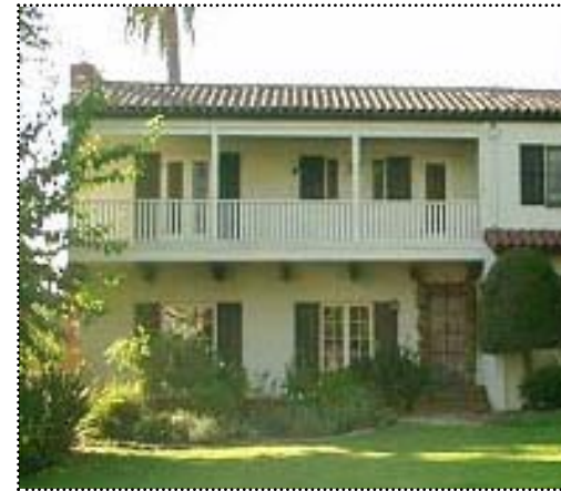
Above: The recessed balcony on the main facade is the primary character-defining feature of the Monterey Revival style.
