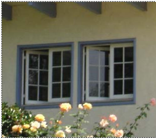
Above: This house has wooden casement windows.
