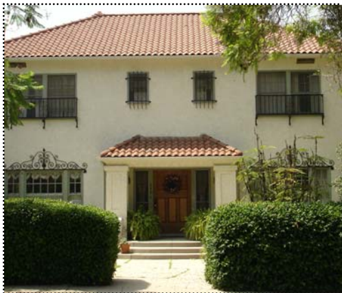
Below: A single-story addition at the sides or rear of this house would be appropriate to the scale and massing of the established structure.
