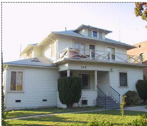
Below: Unusual for the style, this house has a one-story wing on the secondary facade. Both the siding and the pitch of the roof reflect the character-defining features of the main house.
