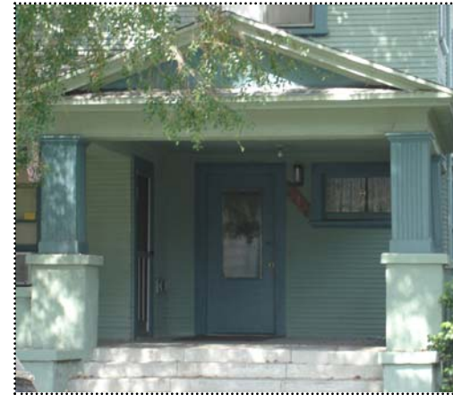
Above: The porch has square piers and a gabled pediment to mark the building's entry.
