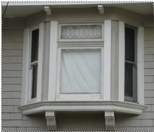
Below: This oriel window has characteristic component parts--wood double-hung sash as well as a stylized fixed upper sash in the center window.
