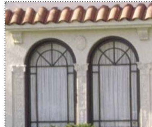
Below: These arched windows on a Spanish Colonial Revival house have decorative muntins and a red tile hood.
