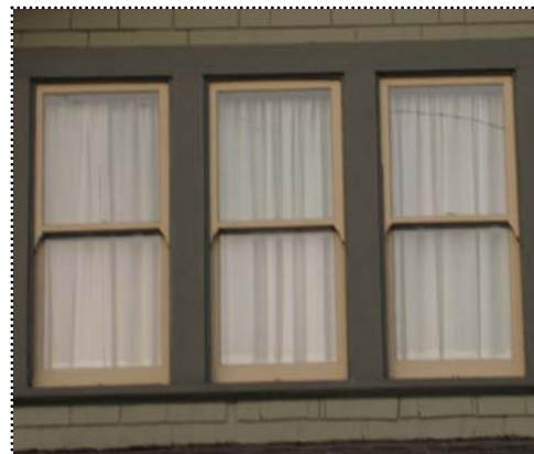
Above: Steel casement windows at building corner Below: Row of wood double-hung 1-over-1
