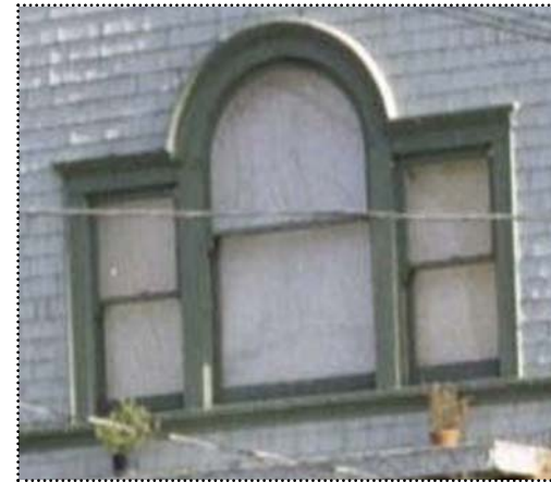
Above: Palladian windows, like the one shown above, have a central larger arched window flanked by two smaller non-arched windows.
